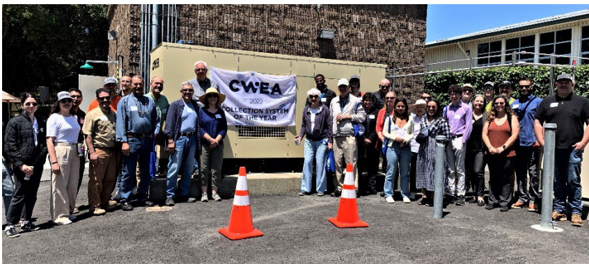
Community members and RVSD staff joined in for a group photo at Pump Station 14 (Larkspur) on July 19.
