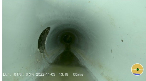
CCTV Footage Inside HDPE Pipe
