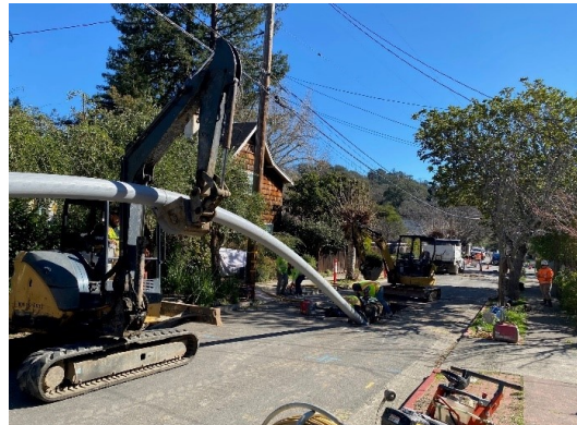
Glosage Installing New HDPE Pipe
